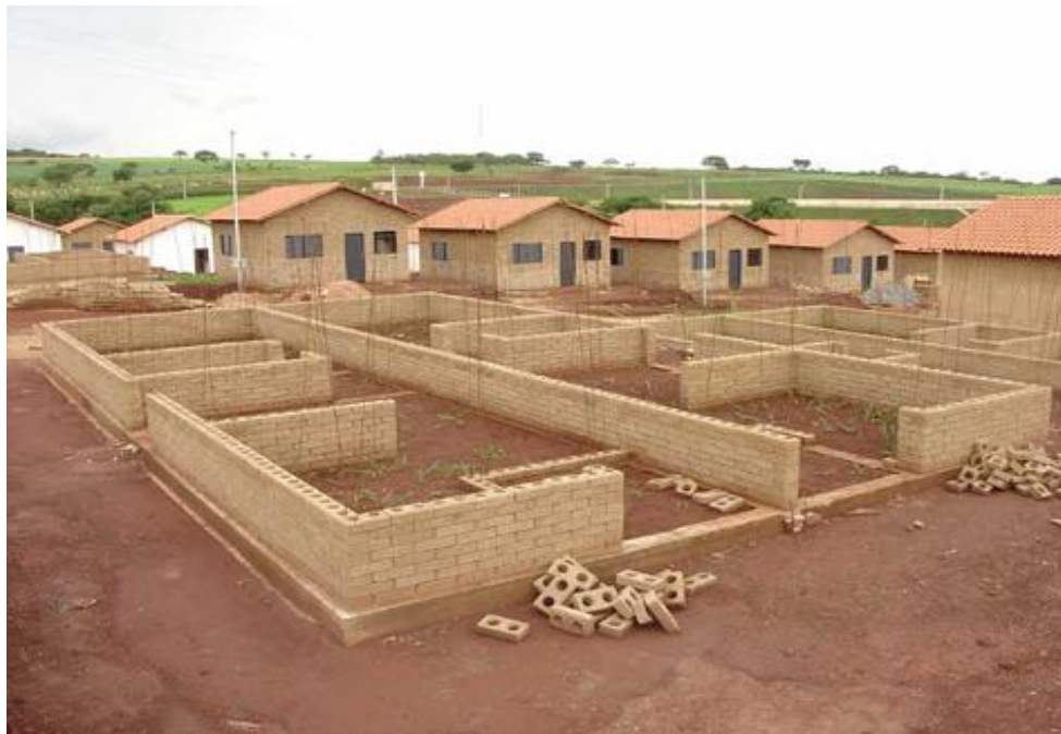
un CHANTIER STABIBLOCK' System
