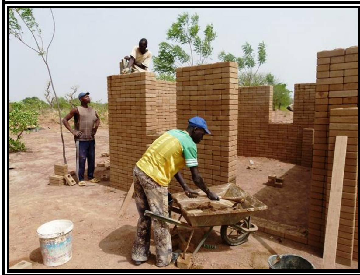
Un CHANTIER STABIBLOCK' System
